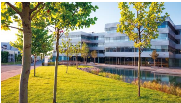
BREEAM Excellent Facility
